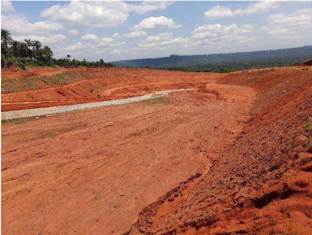
Section view of Urualla erosion site
