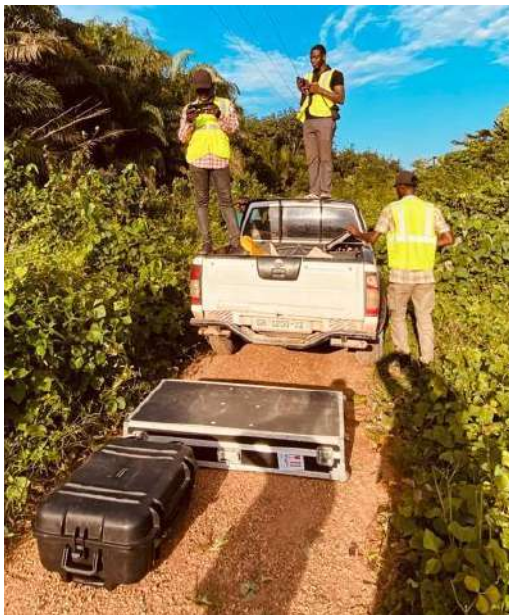
Team preparing the DJI M300 and the YS Mapper LiDAR scanner for LiDAR Scanning
