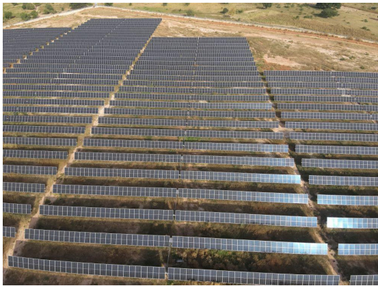
Solar power plant
